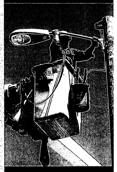
All fixtures feature "full cutoff" technology that offers precise ground coverage while reducing sky glare.
