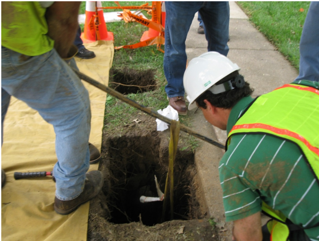
Photograph #5—3-inch main Fusion Inspection (Photograph taken by Staff)
