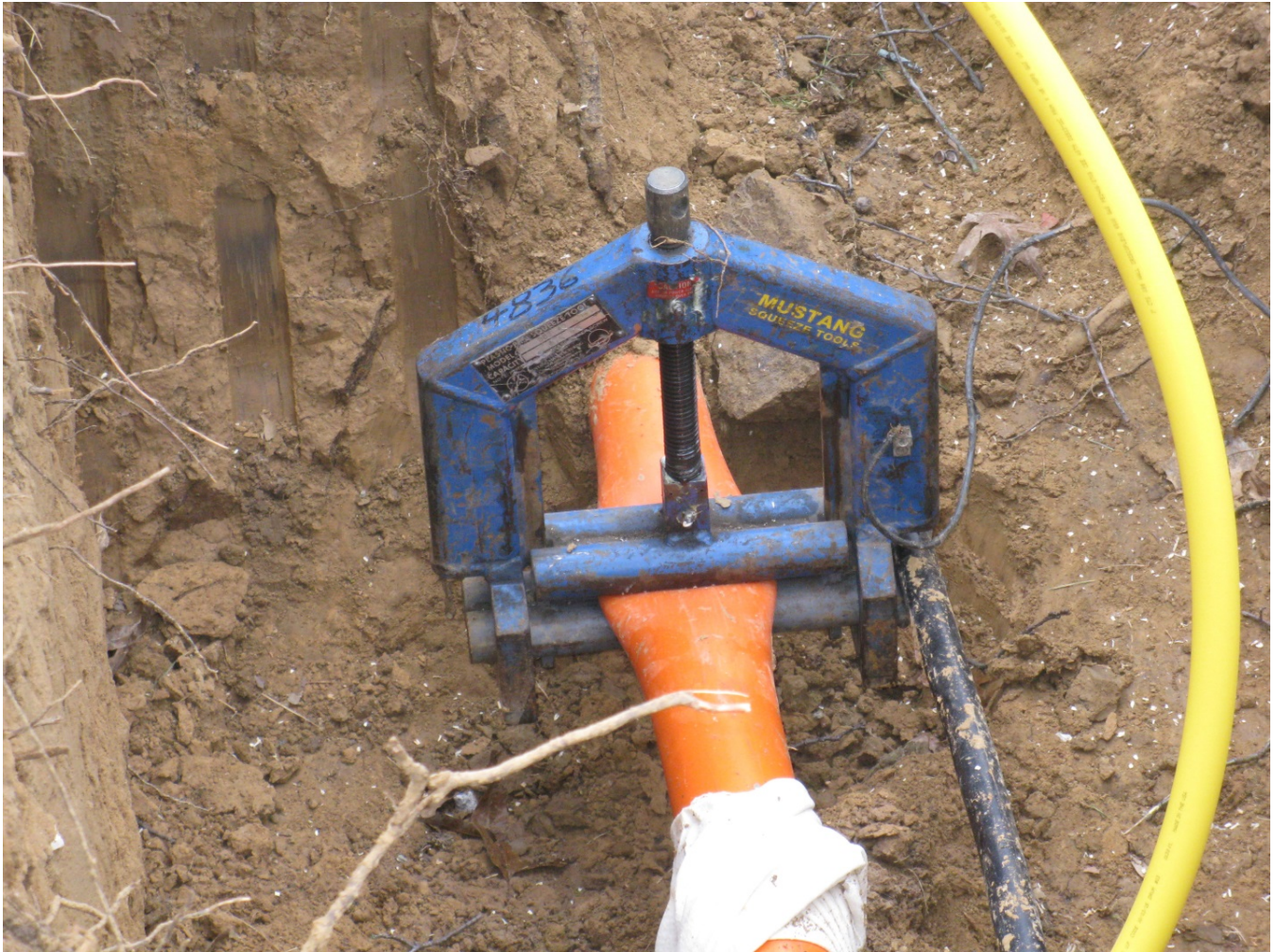
Photograph #17—Viewing the squeeze off location just upstream of the leak location on the main (Photograph taken by Staff).
