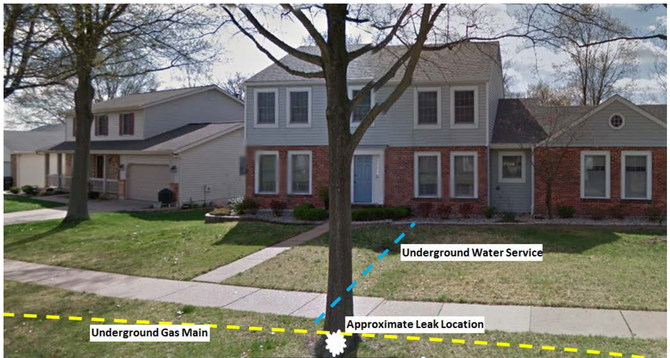
Photograph #2 – The 3-inch PE main and subject butt heat-fusion joint were under this tree (Photograph by google maps).
