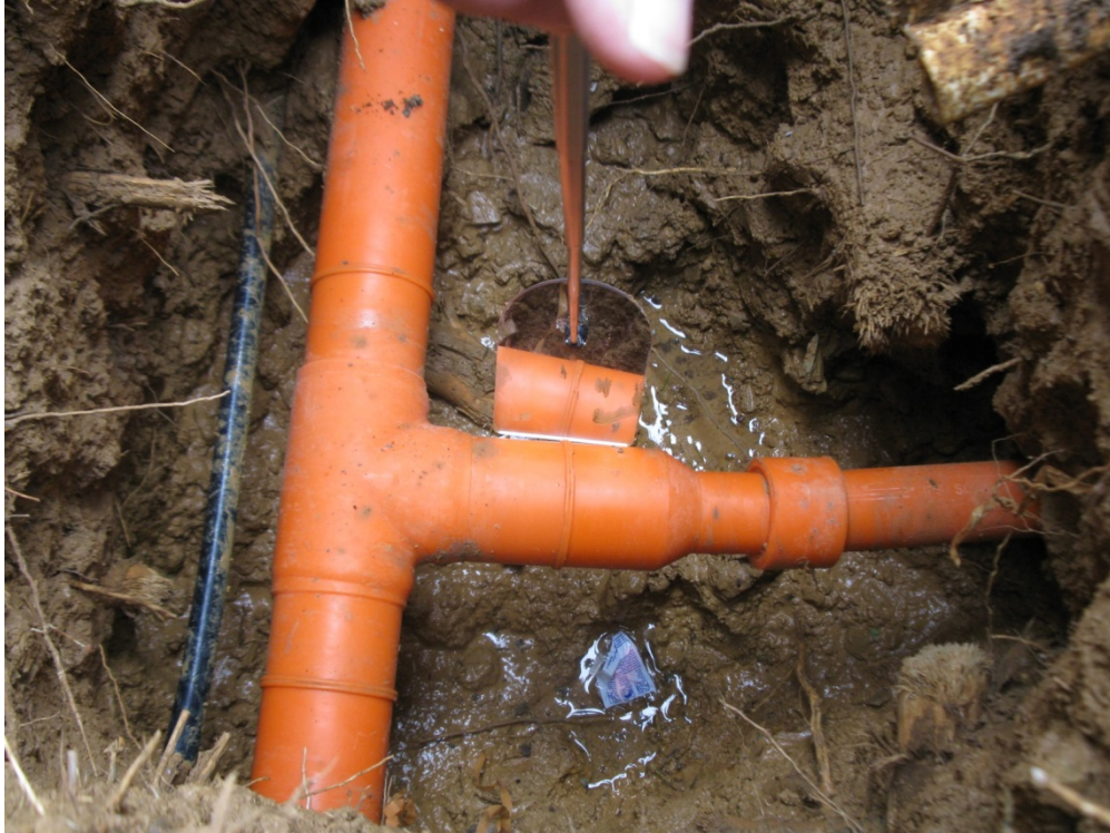
Photograph #4—3-in Main Fusion inspection (Photograph taken by Staff)
