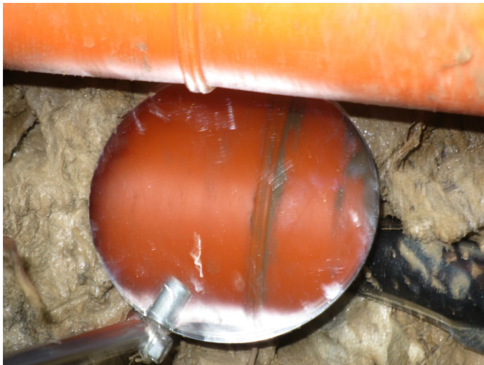
Photograph #3—3-inch main fusion inspection (Photograph taken by Staff)
