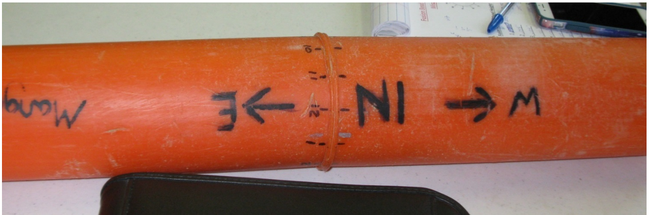
Photograph #8—3-inch main segment (Photograph taken by Staff)
