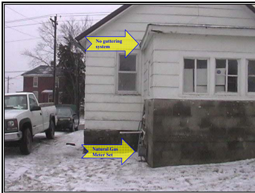
Photograph 1 Looking south at the north side of 715 E. 4 th Street. The natural gas meter set is located on the east wall of the mud room. Observe the roof overhang in relation to the location of the natural gas meter set. No guttering system was installed on any portion of the roof.
