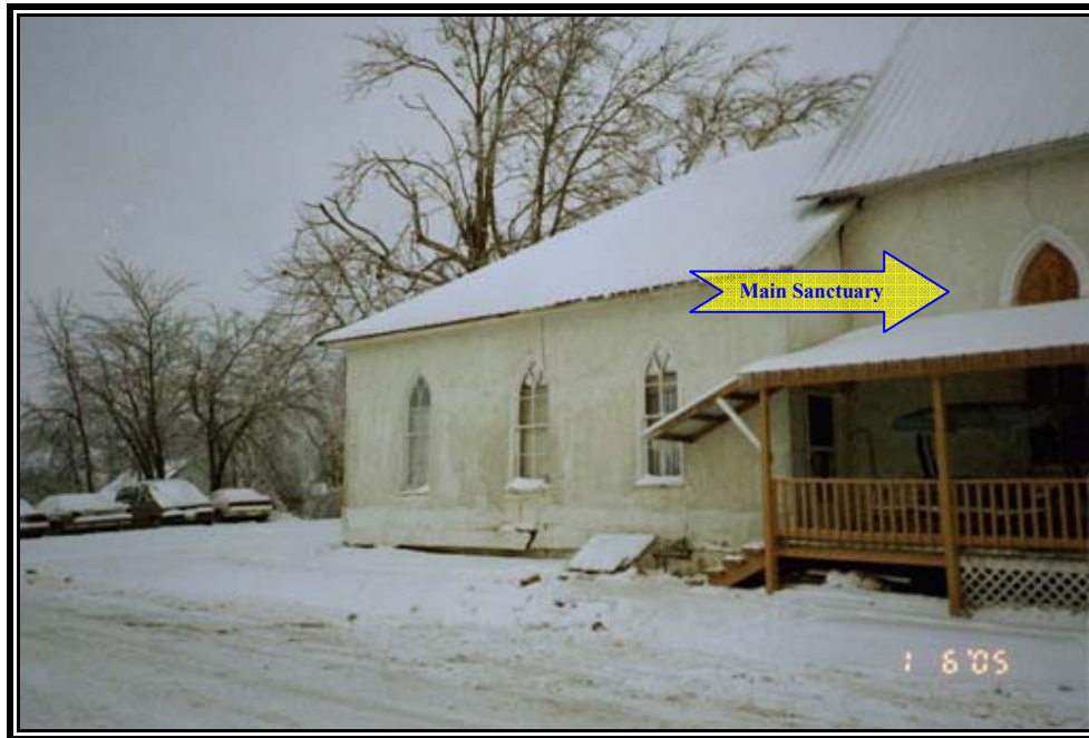
Photograph 5 This view is looking to the northeast at the west side of 1328 Main Street. The street seen in this photograph is 14 th Street which runs north and south. The entire roof structure consisted of a metal roof. Note how the roof overhang from the main sanctuary portion of the residence drained onto the below roof for the wooden porch area.
