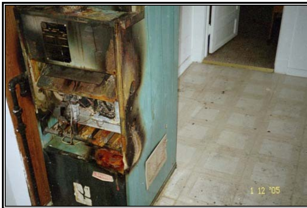
Photograph 6 View of the natural gas furnace that was located in a room along the west side of the residence. This room was located to the west of the dining room area. Note the severe fire damage to the main burner assemblies, as well as, the top and side portions.
