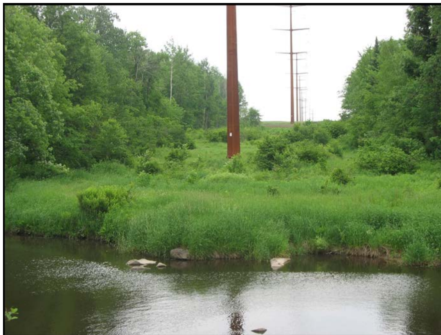
Figure 6 Restored River Bank Following Construction
