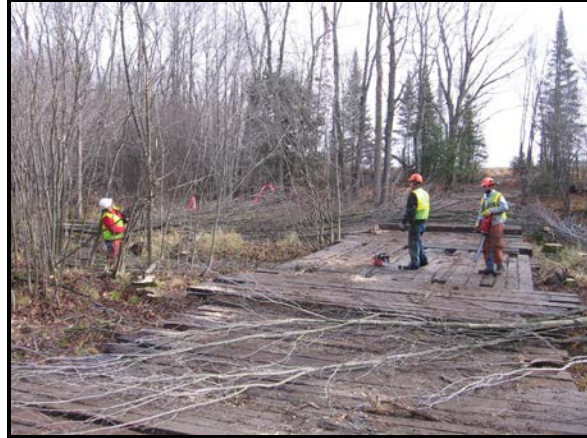
Figure 10 Hand Clearing Channel
