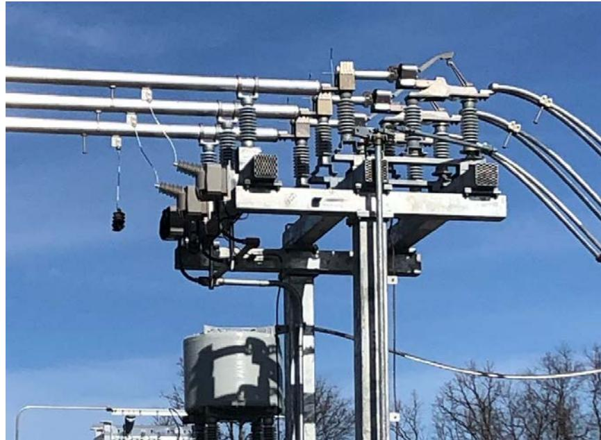
Picture 1. Failed voltage transformer on far medium voltage bus resulted in a plant outage on December 26<sup>th</sup>.
