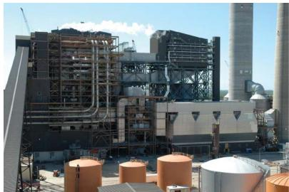
**2. Duplicated design.** The design of the air quality control systems for the two units was very similar. On latan 1, the selective catalytic reduction (SCR) system was placed away from the unit because of retrofit space constraints; for latan 2, the SCR system was part of the integral design. Otherwise, the same catalyst type and size was used, and both boxes are able to hold four layers, although only two layers are currently used on each unit. *Courtesy: KCP&L*
