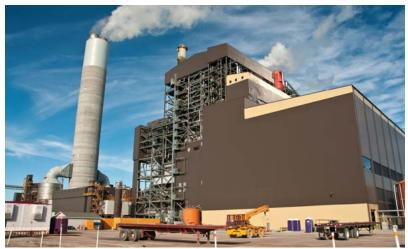
**4. Combined stack.** The two units' wet scrubber vessels are located on opposite sides of the new combined stack. Note that the SCR system is integrated into the structure of latan 2, unlike at latan 1, shown in Figure 2. *Courtesy: KCP&L*
