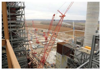
**6. Tight site.** The project team was responsible for managing a very constrained work site where multiple contractors were working on the air quality control equipment upgrades on latan 1 at the same time as latan 2 was under construction. At the project peak, 4,000 workers were on site. *Courtesy: KCP&L*
