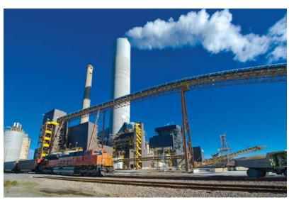
**3. Carrying coal.** Coal is delivered to each of the two units via a common, redundant conveyor system. The conveyor is enclosed with dust collectors, ensuring no fugitive emissions occur. *Courtesy: KCP&L*
