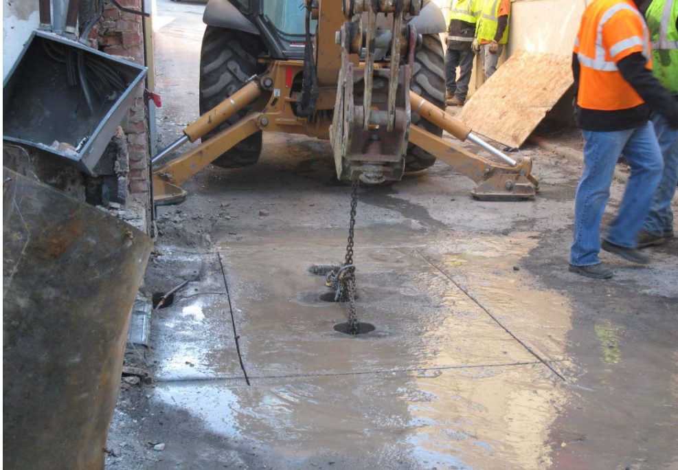
Photograph #5 – Slab of pavement to be removed in the alley near the northeast corner of JJ's Restaurant containing potholes 3, 4 and 5 (Staff Photo)
