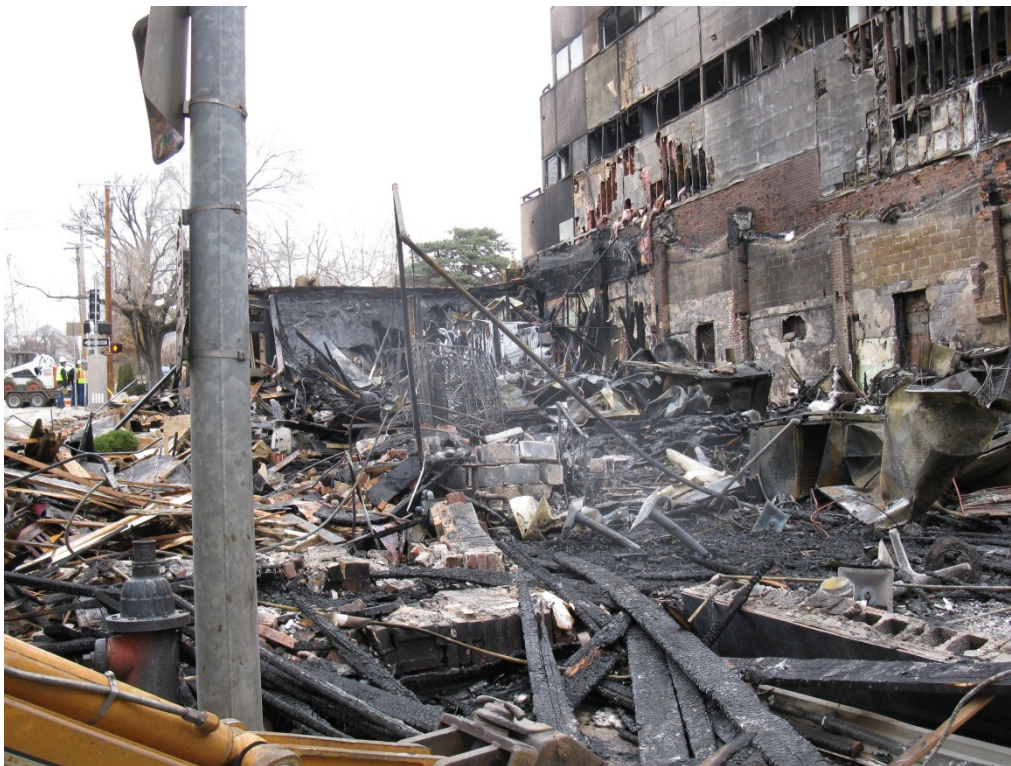
Photograph #8 – Damage and debris from what remains of JJ's Restaurant facing west (Staff Photo)
