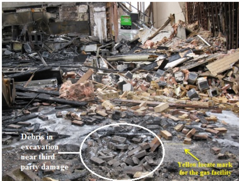
Photograph #14 – Debris in the alley between JJ's Restaurant and the House of Elan facing north (Staff Photo)
