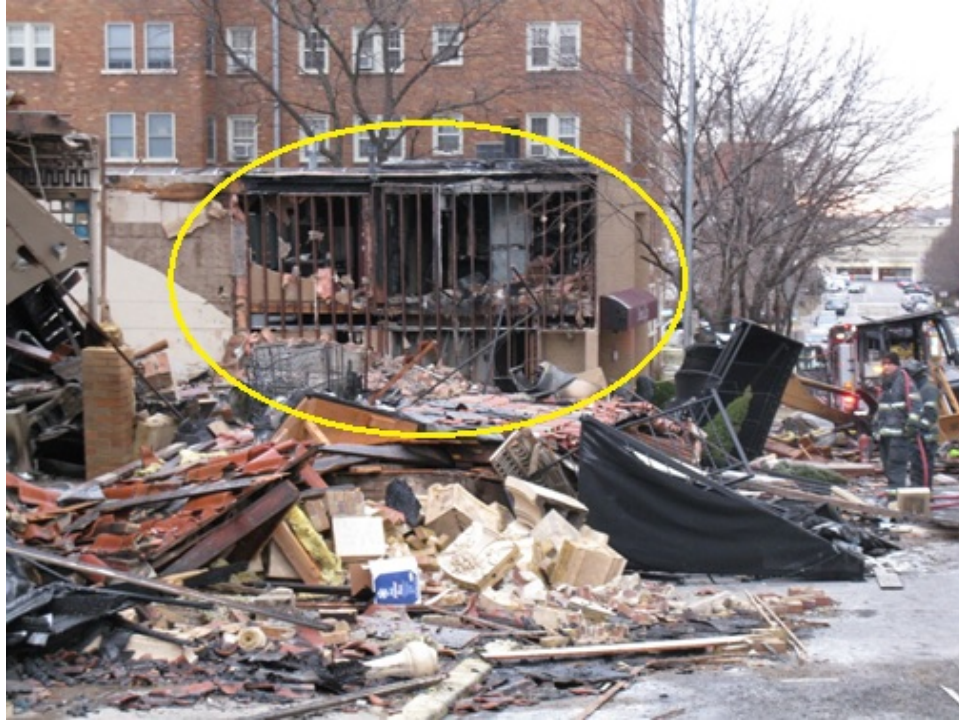
Photograph #9 – The west side of the House of Elan sustained significant damage during the explosion and subsequent fire. Debris from JJ's Restaurant is shown in the foreground. This Photograph was taken looking east down W. 48 th Street (Staff Photo).
