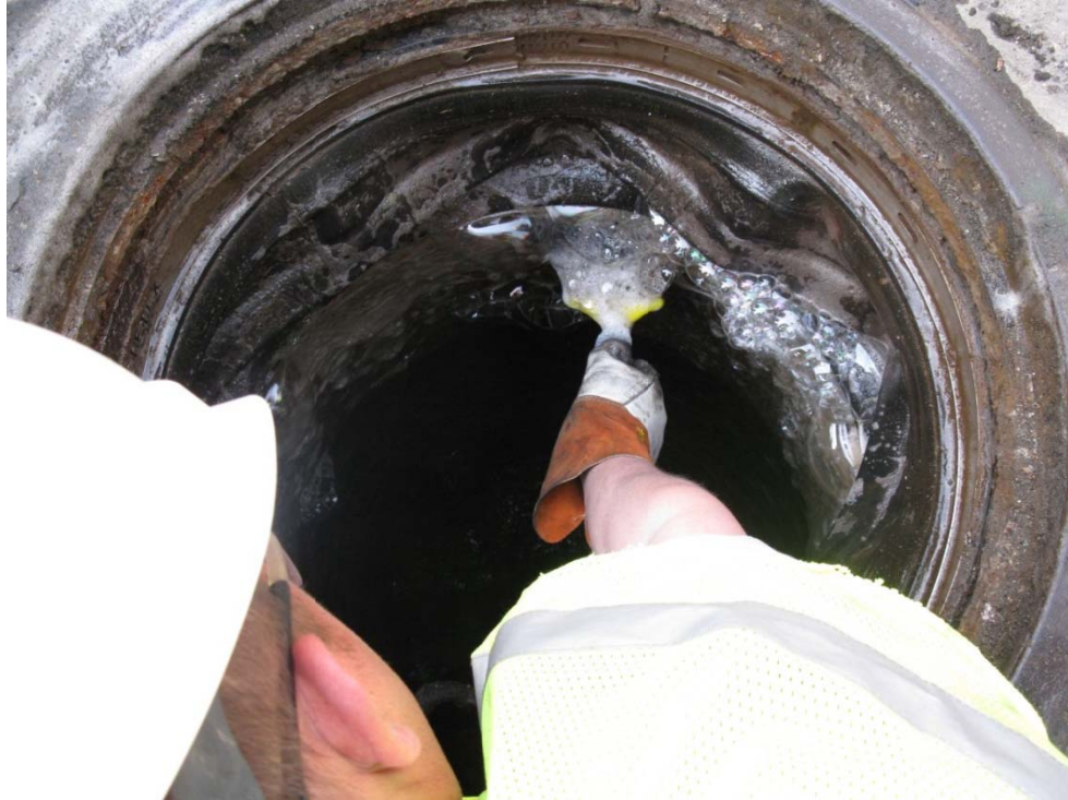
Photograph #19 – Soap test in the sanitary sewer manhole across from the alley between JJ’s Restaurant and the House of Elan near the third-party damage (Staff Photo)
