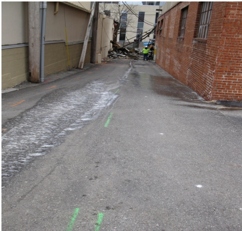
Photograph #3 – Pothole #6 is shown between the line of yellow marks (circled in yellow) and the line of red marks (circled in red) near the approximate area of the damaged main. The white dots represent the bore path. The “37” written to the left (south) of the pothole indicates a drill bit depth of approximately 37 inches, while the “3” on the right (north) side of the pothole represents a drill bit depth of approximately 3 feet. (Provided by MGE)
