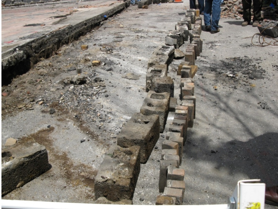
Photograph #25 – Cinder blocks and bricks removed from the east wall of JJ's Restaurant to expose void spaces beneath the floor slab. (Staff Photo)
