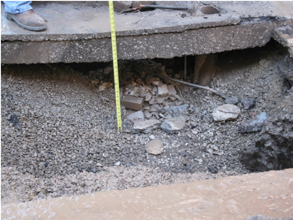
Photograph #5 – Slab of pavement to be removed in the alley near the northeast corner of JJ's Restaurant containing potholes 3, 4 and 5 (Staff Photo)
