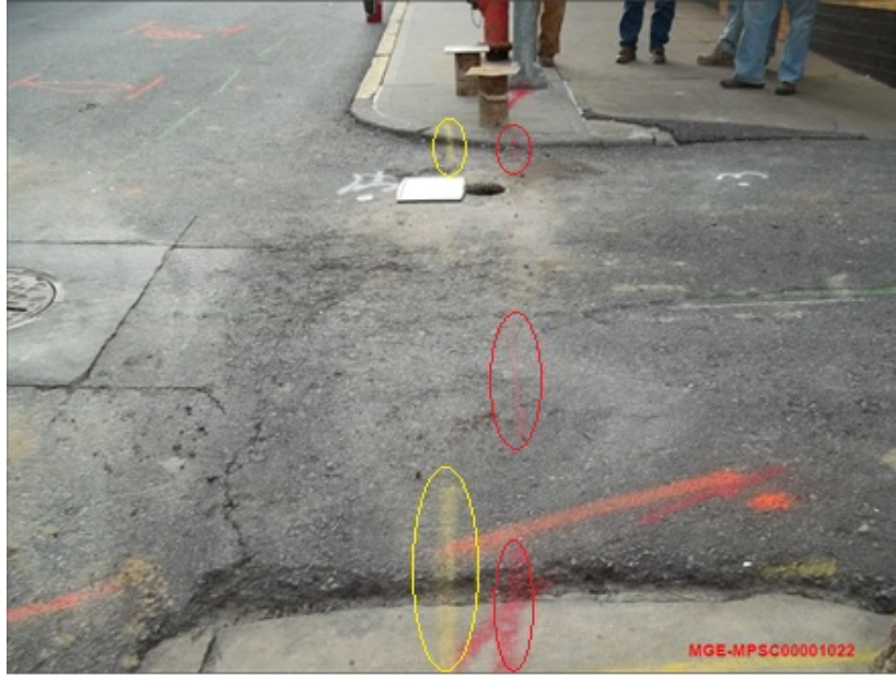
Photograph #3 – Pothole #6 is shown between the line of yellow marks (circled in yellow) and the line of red marks (circled in red) near the approximate area of the damaged main. The white dots represent the bore path. The “37” written to the left (south) of the pothole indicates a drill bit depth of approximately 37 inches, while the “3” on the right (north) side of the pothole represents a drill bit depth of approximately 3 feet. (Provided by MGE)
