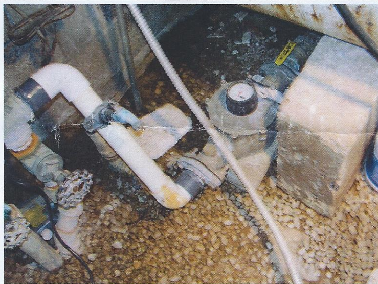
Photo #: 3 By: Fred Mashburn Facility: Roy-L Utilities Permit: MO6251710 Location: Well #2, well house interior. Description: Well #2 Master Meter.
