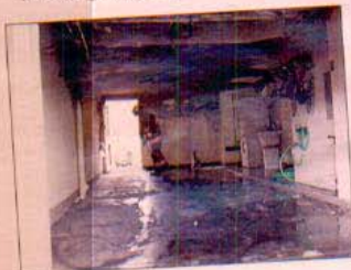
The wiring in the ceiling, which didn't melt, shows how sprinklers controlled the fire.
