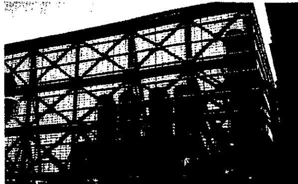
2. Architectural screen shields generating equipment from public view, but allows the plant to "breathe"
