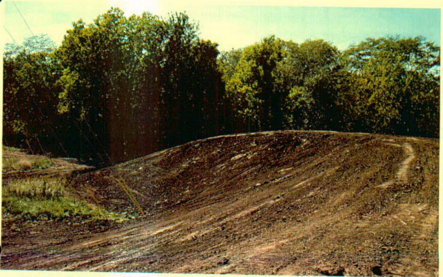
Construction of Berm - On Aquila Property
