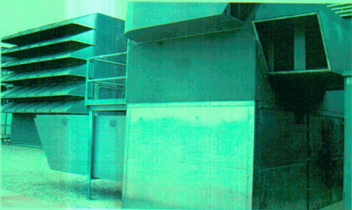
Photo No. 4.2-3 – Regulating Station Gas Vent Silencer
