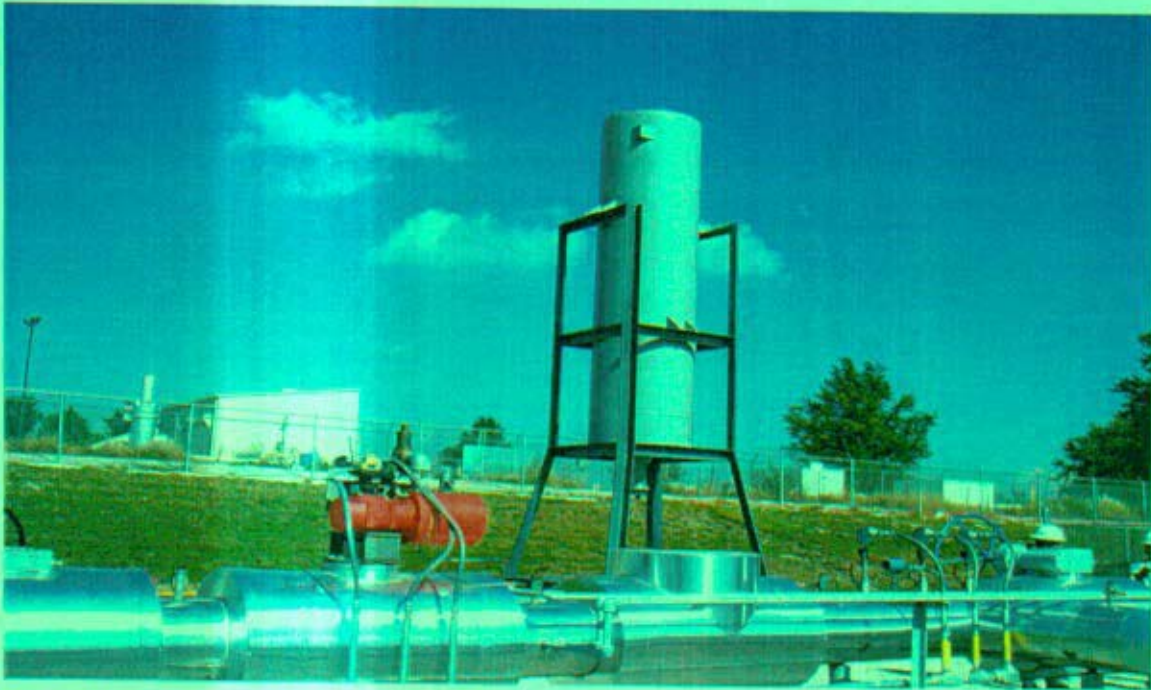
Photo No. 4.2-3 – Regulating Station Gas Vent Silencer
