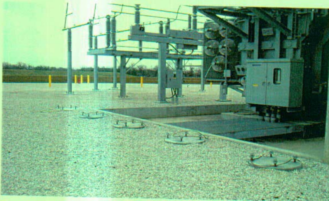
Photo No. 4.2-6 – Generator Step Up Transformer Sound Wall Foundations
