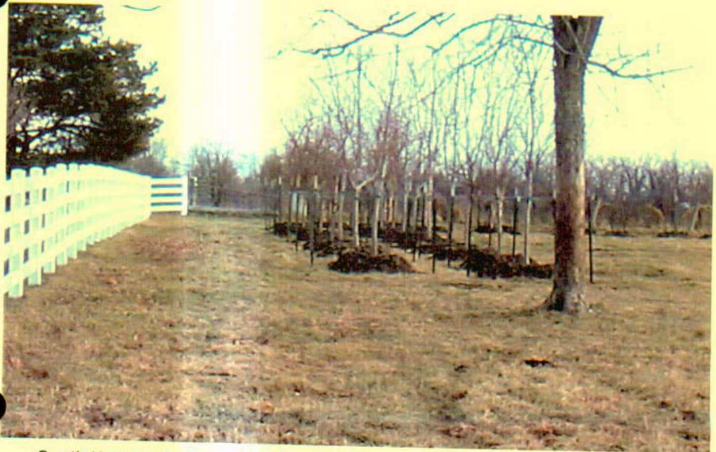
South Harper Road - on Aquila Property
