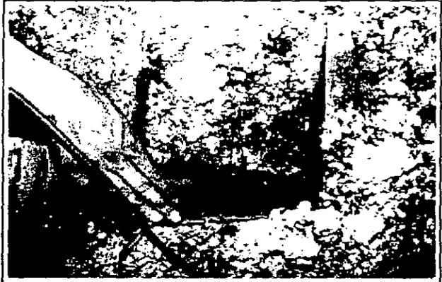
**Interior walls open to attics are commonplace—and must be sealed to prevent thermal siphoning. If this hole is not sealed during weatherization, the interior wall below is likely to be much colder in the winter than exterior insulated walls.**
