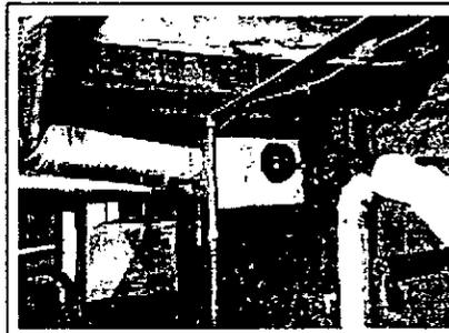
Holes like these in supply ducts can be quite wasteful--yet they can be repaired quickly and cost effectively.
