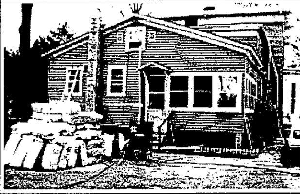
Installing cellulose at high density has been found to be a powerful technique for installing insulation and achieving air sealing at the same time. Many crews find that the infiltration rates of some houses can be cut in half without using a tube of caulk. The secret is careful installation of high-density cellulose in wall cavities (and other places where it really counts) with a tube inserted directly where the insulation needs to go--and using power blowing machines to pack it in tightly.
