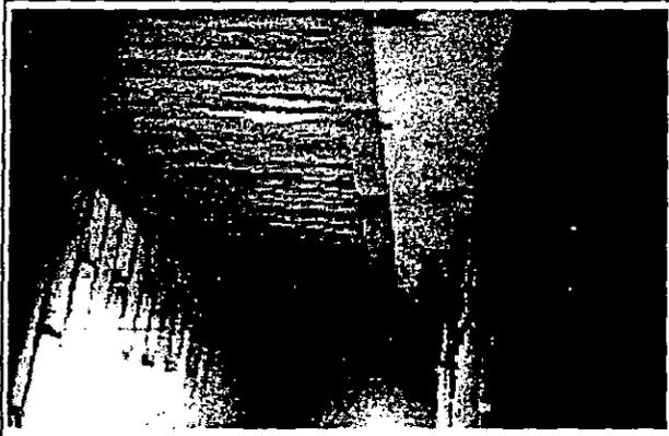
**This space between the chimney interior framing is completely open to the attic. Sealing this at the level of the attic insulation is likely to save more energy than replacing every window in the dwelling. An experienced weatherization crew technician can thoroughly (and safely) seal this opening in 15 minutes with a material cost of \$4.**
