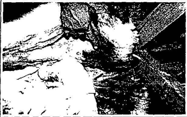
**This is a 12-inch fiberglass batt that has been on top of a small crack in the ceiling below for only one winter. The dirt is from the passing of massive amounts of air driven by stack-effect exfiltration.**
