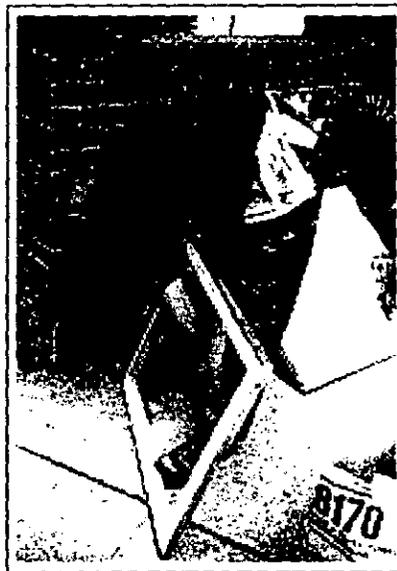
Glass replacement is inevitably time consuming but necessary. Most agencies rebuild the sash to ensure good air sealing.
