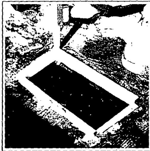
The interface between the riser in a supply duct and the floor of a mobile home is frequently found to be a source of air leaks, both when the furnace fan is on and when it is not. Here a technician in Indiana uses a technique his agency developed to achieve a tight, lifelong seal.
