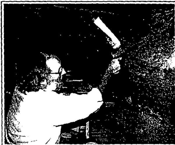
Air sealing at sill plate with foam. This infiltration-stopping measure is necessary with most weatherization jobs.
