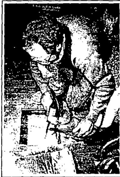
**Single-component foams in conjunction with rigid board stock cut to fit attic openings achieve tight, long-lasting attic sealing.**
