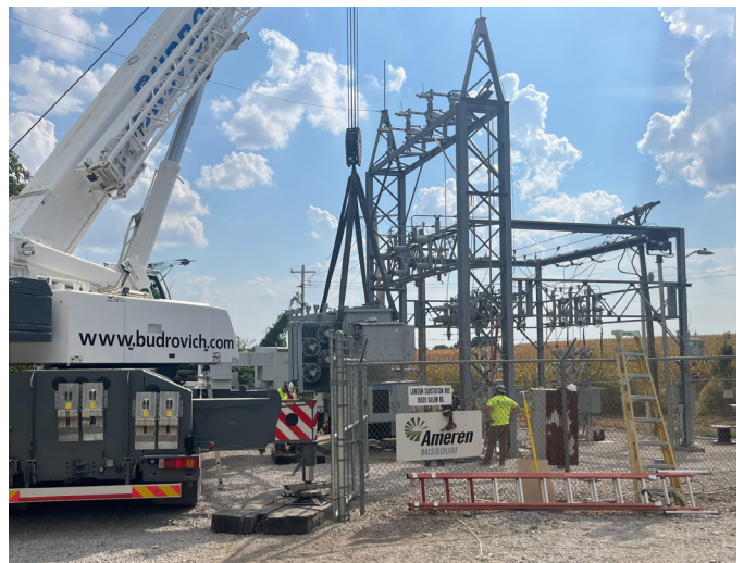
An upgraded substation under construction in St. Louis.
