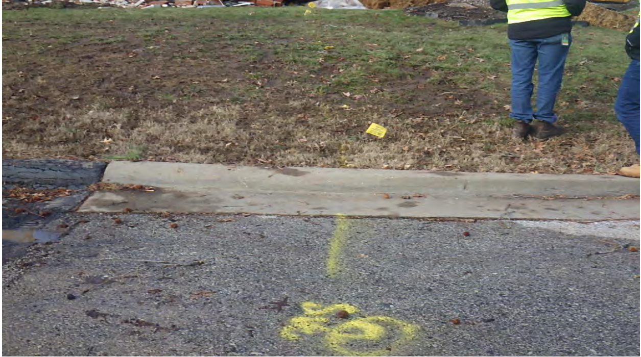
Figure 2 – USIC Natural Gas Locate Made Prior to Incident.
