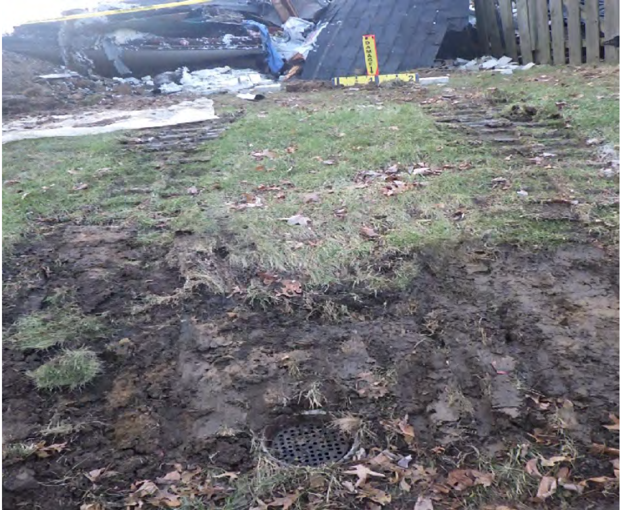
Figure 12 – Excavator’s work site
