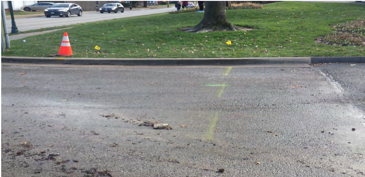
Figure 3 – USIC Natural gas service locate
