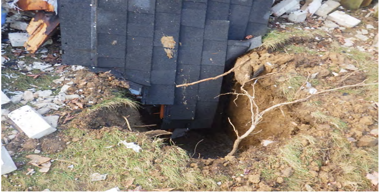
Figure 4 – Excavation Made Prior to Incident
