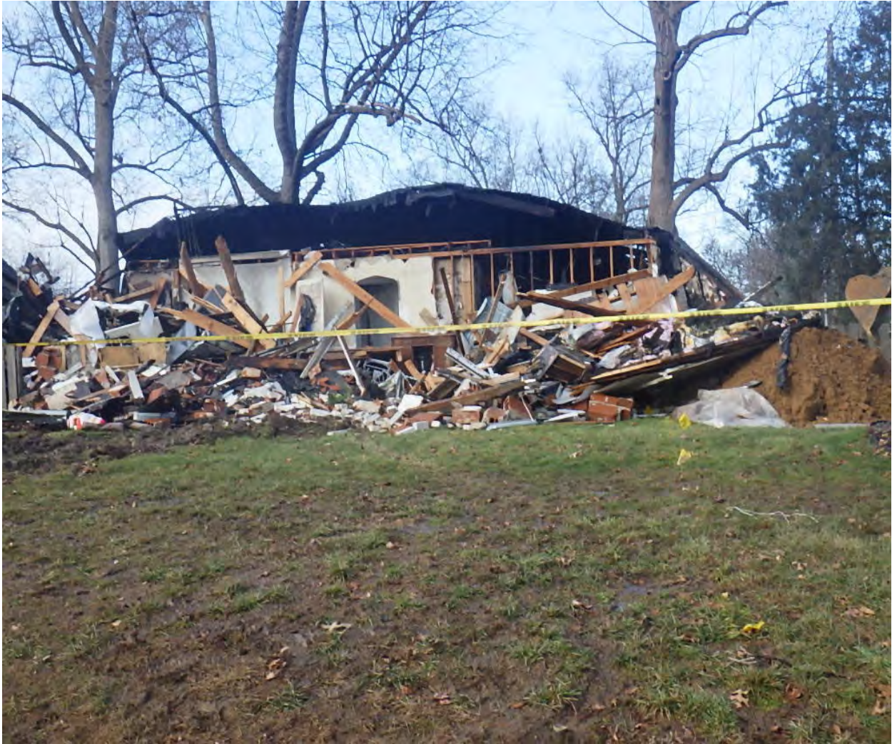
Figure 1 - Front of 895 Glen Elm Drive Following the Explosion.
