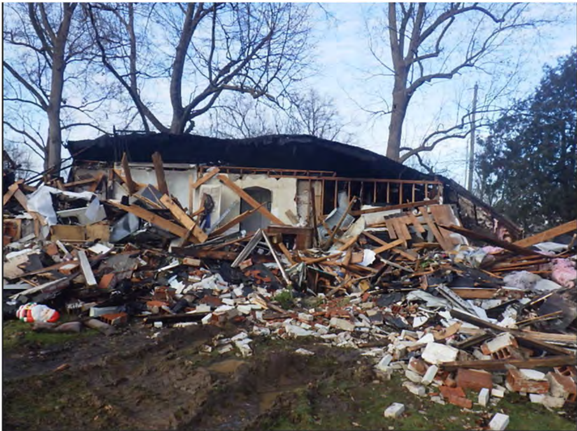
Figure 3: Residence at 895 Glen Elm Dr. on January 3, 2025, following explosion. Photograph was taken from Glen Elm Dr. looking North. (Source: Staff Photograph)
