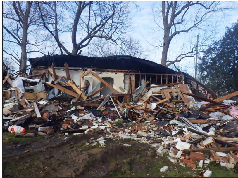
Figure 2: Residence at 895 Glen Elm Dr. on January 3, 2025, following explosion. Photograph was taken from Glen Elm Dr. looking North. (Source: Staff Photograph)
