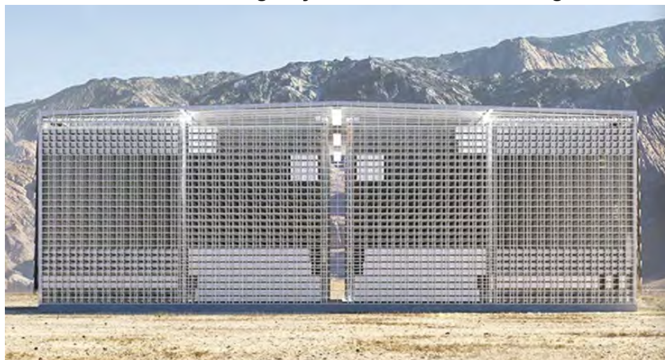
Figure 6.11 Concrete Block Storage System – Blocks in a Large Modular Grid 16
