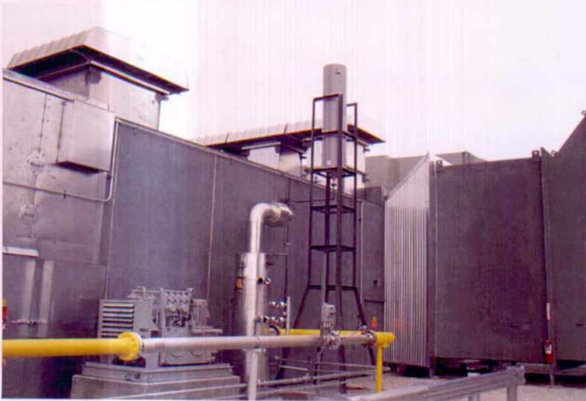
Photo No. 4.2-2 – Turbine Gas Vent Silencer
