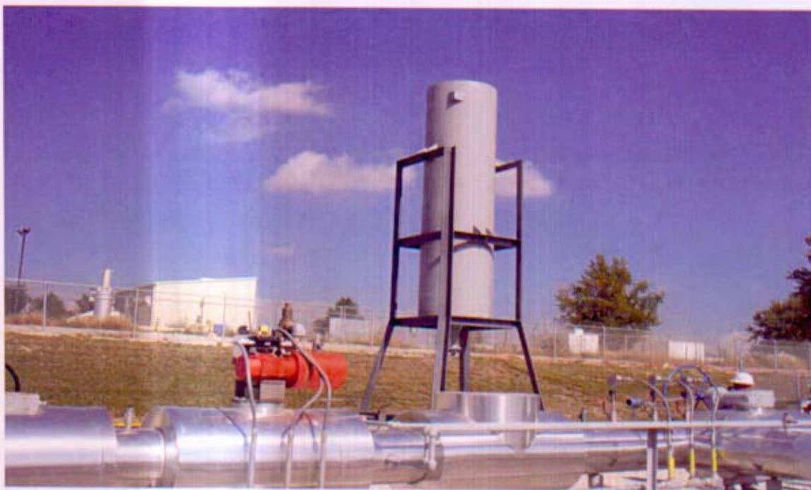
Photo No. 4.2-3 – Regulating Station Gas Vent Silencer
