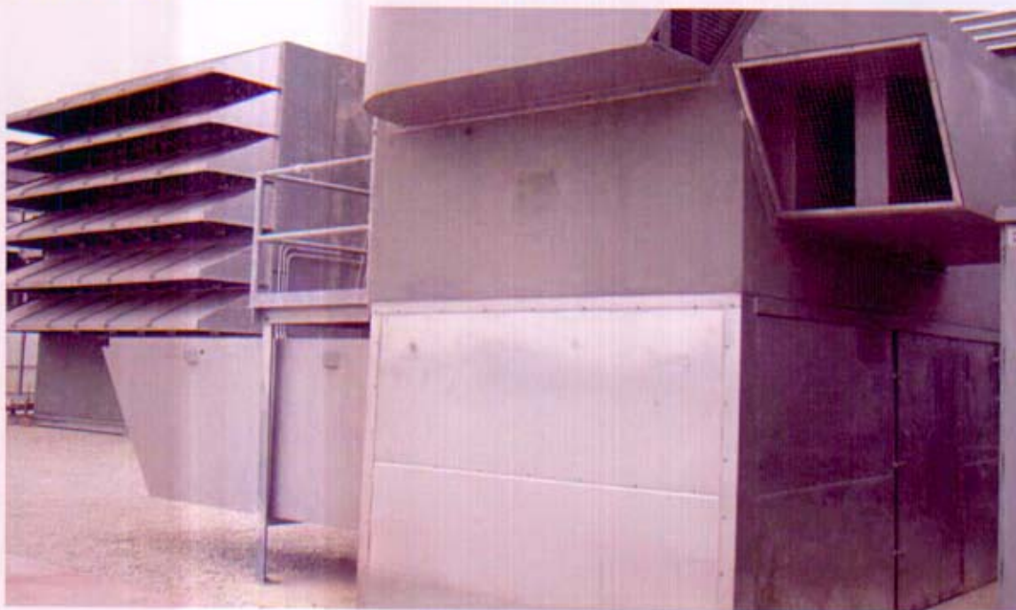
Photo No. 4.2-3 – Regulating Station Gas Vent Silencer
