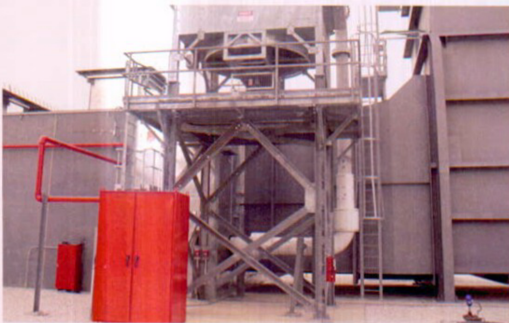
Photo No. 11 - Combustion Turbine Enclosure FM-200 Cabinet
