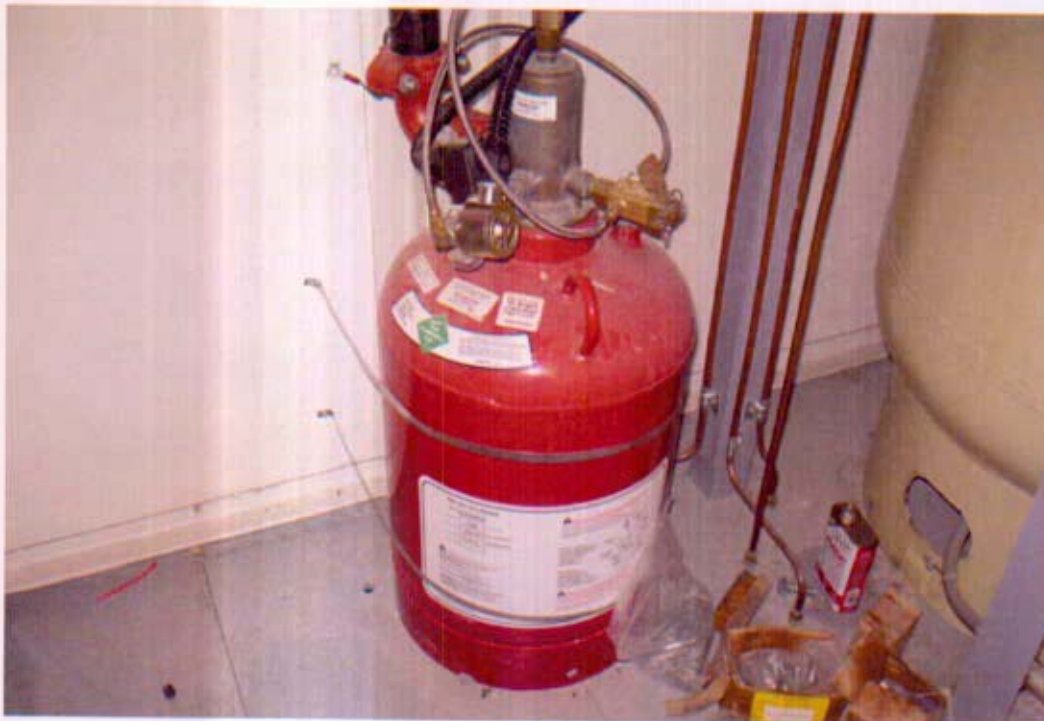
Photo No. 13 - Mechanical Package FM-200 Bottle.
