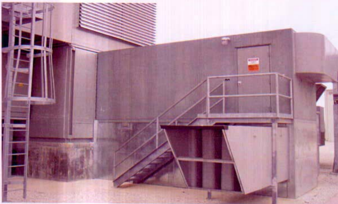
Photo No. 4.2-5 – Starting motor package ventilation silencer
