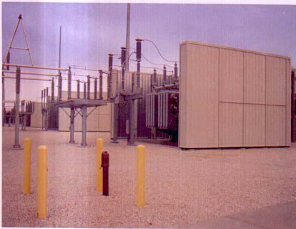
Photo No. 4.2-9 – Generator Step-Up Transformer Sound Walls
