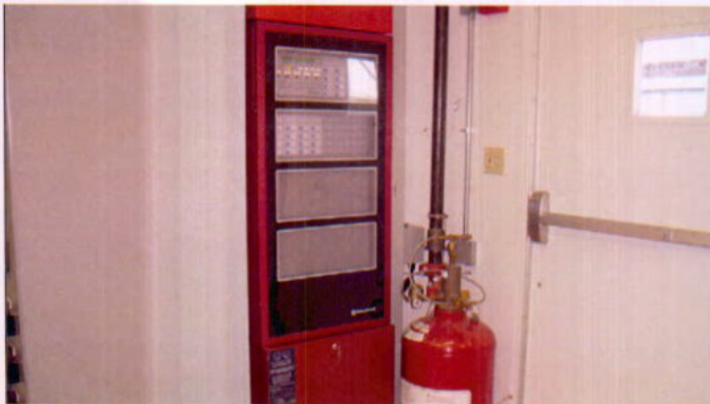
Photo No. 10 - Fire Suppression System Control Panel, located in Electrical Package.
