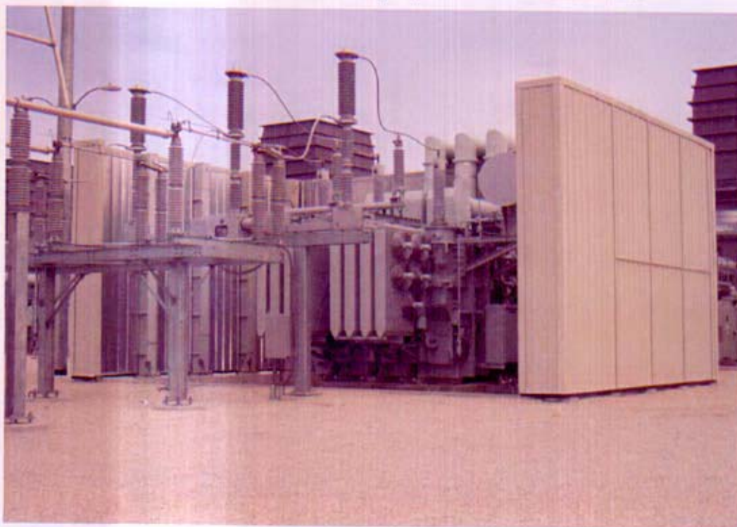
Photo No. 4.2-10 – Generator Step-Up Transformer Sound Walls
