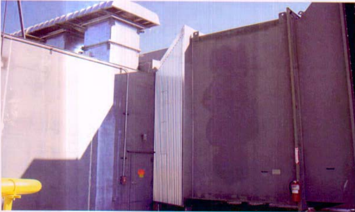
Photo No. 4.2 -1 – Acoustic Lagging on Air Inlet Transition
