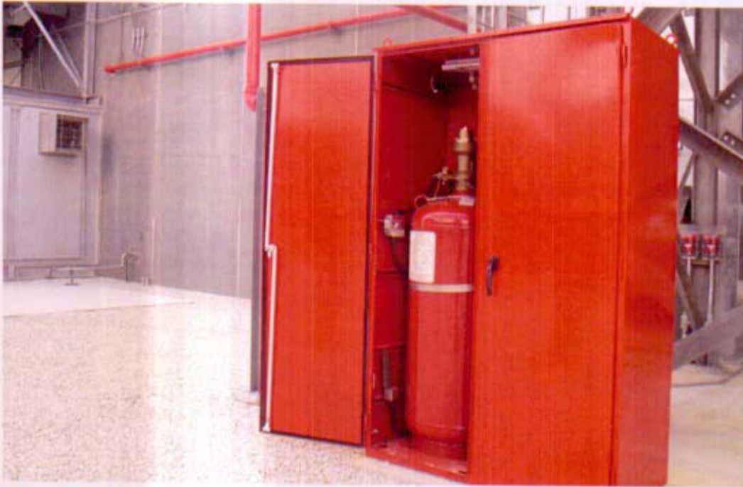
Photo No. 12 - Combustion Turbine Enclosure with FM-200 Bottle.
